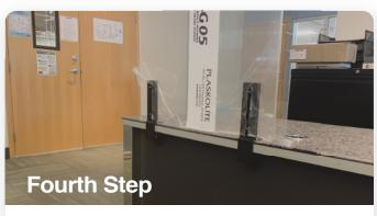
Carefully position the completed assembly onto the table top.
